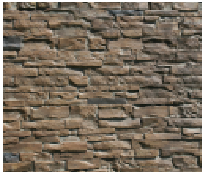
CONCRETE WALLS AND PARTITIONS (LEFT AND RIGHT)
